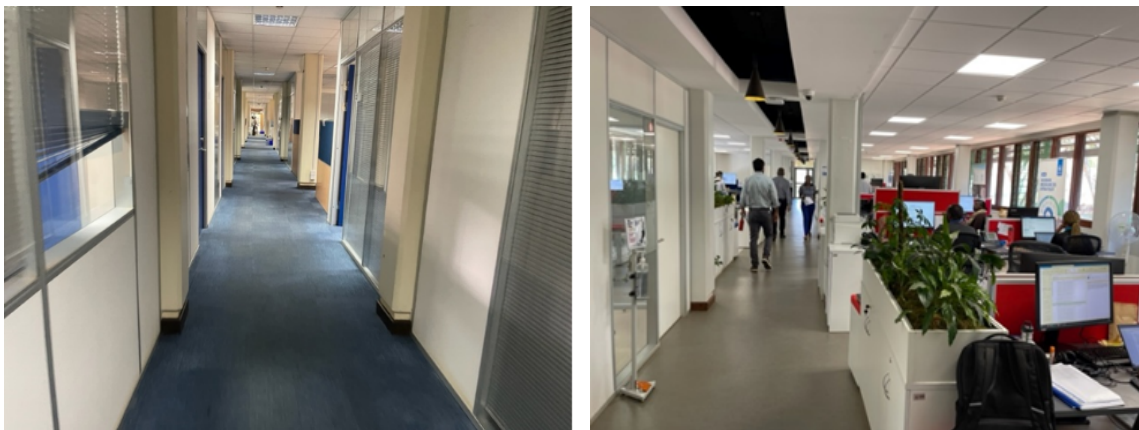
Figure 1: Before and after renovation of office block
