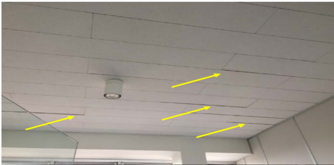
Photo 3: Shaky ceiling due to the impact of a sandstorm
