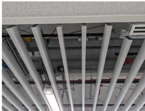
Picture 4 Ceiling on completed floor
