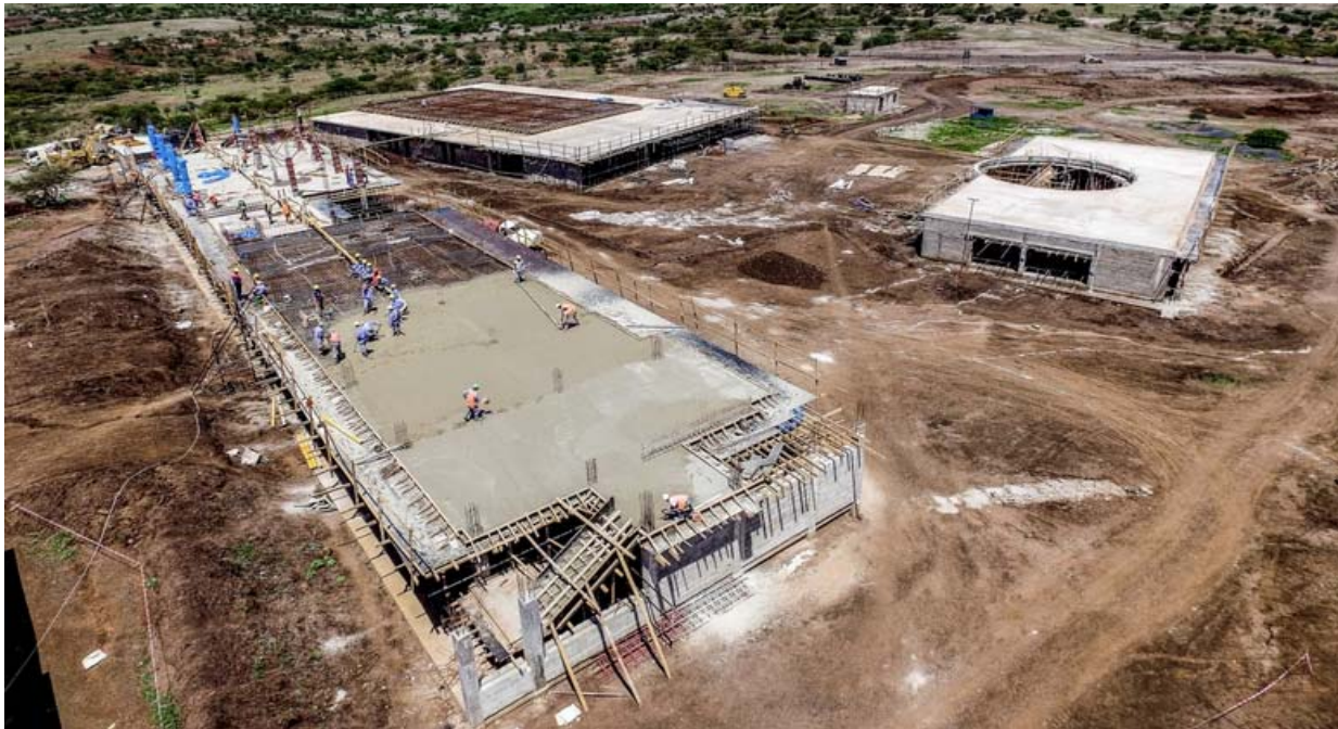
Picture 1: View of the construction site in Arusha (31 December 2015)
